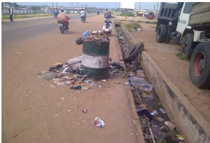
Plate 4. Waste disposal in drainages.
