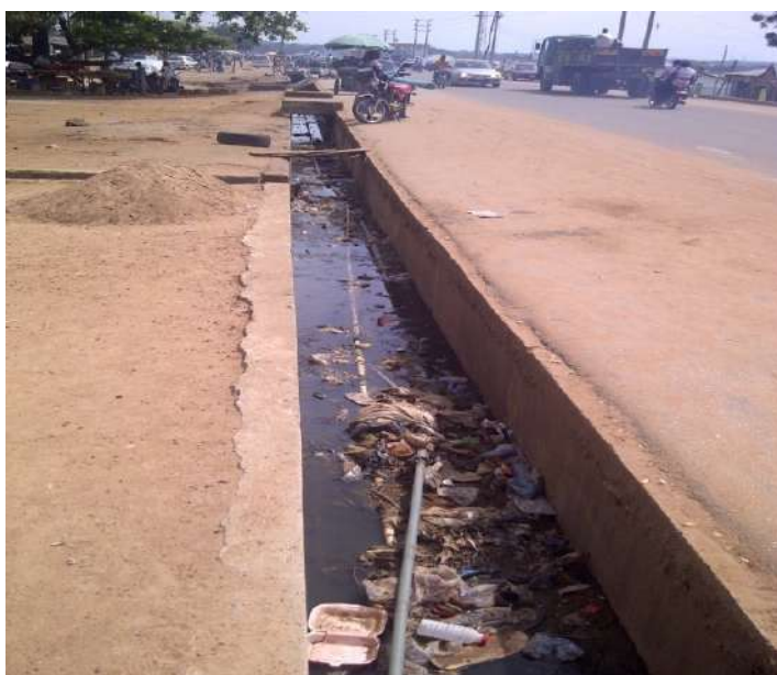
Plate 2. Water pipes laid in drainage.
